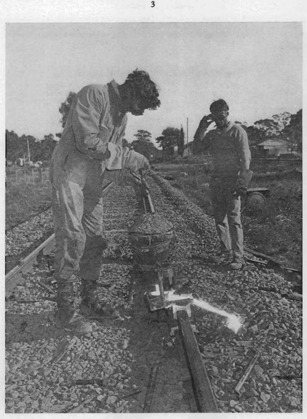
Thermit welding on the standard gauge track between Melbourne and Albury.
